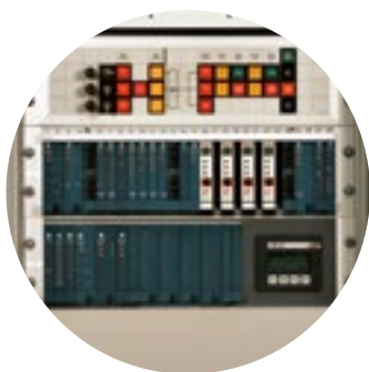
Typical logic solver panel.
