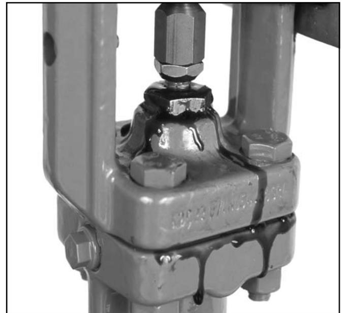
**Figure 3: Ineffective packing systems allow process leakage**
